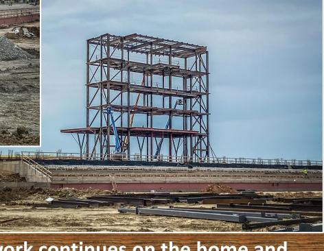
Structural work continues on the home and visitor bleachers and press box. CMU block is being installed in the fieldhouse and is finishing up in the multi-purpose center.
